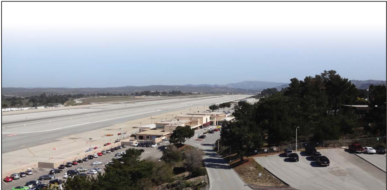
Monterey Regional Airport showing terminal, scheduled for replacement.
