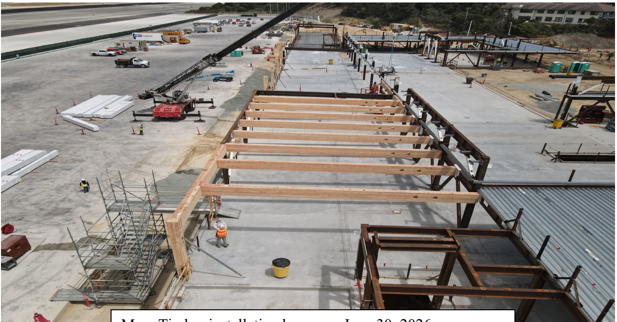
Mass Timber installation began on June 30, 2026
