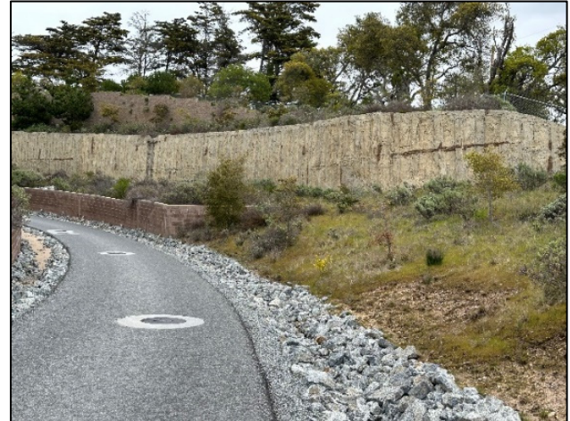
Retaining wall east of vehicle service road
