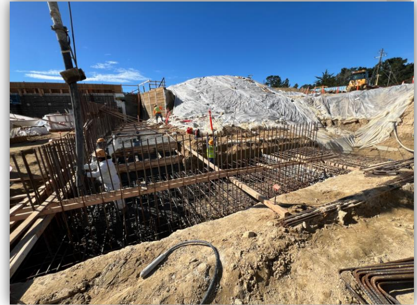
Overcoming weather – 1 week later, place Concrete
