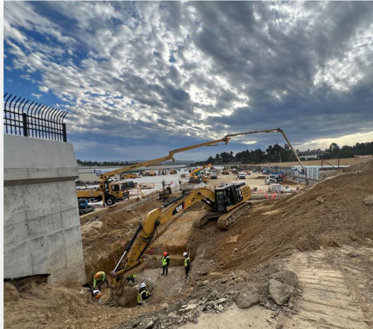
Foundation excavation concrete placement
