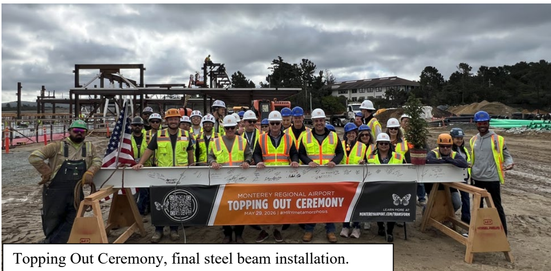
The installation of the steel frame
