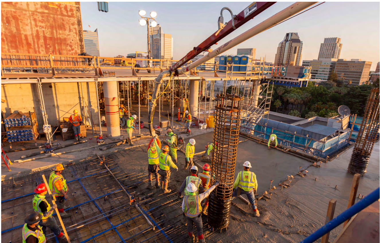
Our self-performing concrete crews on a recent Northern California project
