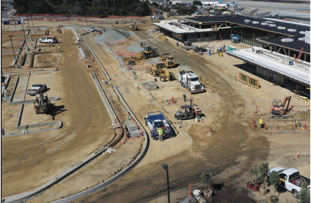
Installation of the premium parking and front curb began in September 2026
